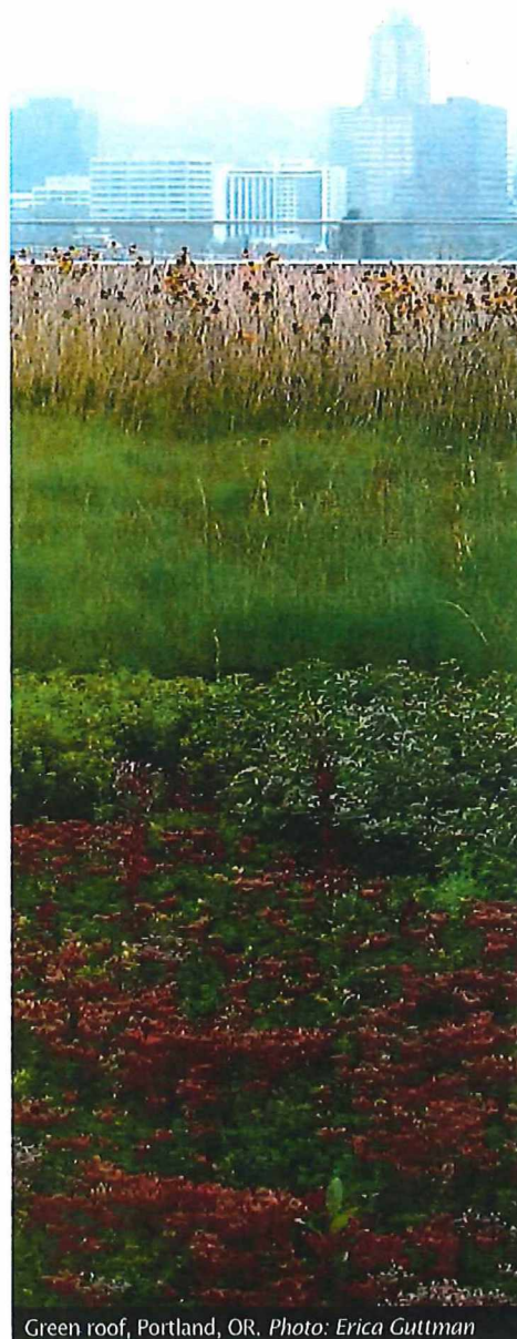
Green roof, Portland, OR. Photo: Erica Guttman
